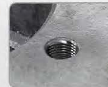
6. Thread is repaired and ready to use
